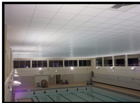
After – new suspended ceiling system lowered by 3.0m
