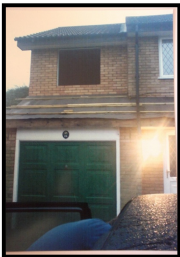
Front view of first floor extension (above existing garage)
