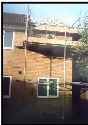
Rear view of first floor extension (above existing utility room)
